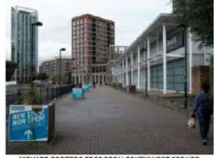
VIEW TO PORTERS EDGE FROM SOUTHWEST CORNER
