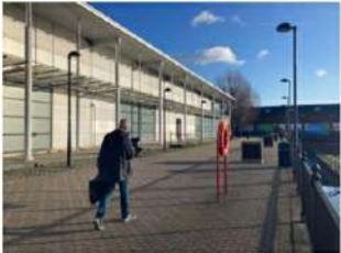
EXISTING BUILDING FROM DOCK EDGE
