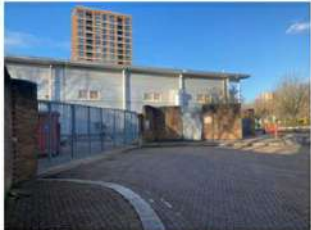
EXISTING SERVICING ACCESS
